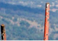
Lightning strike erosion on the lightning arrestor
