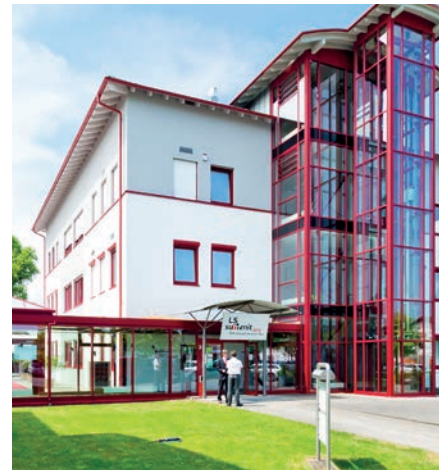
LS telcom Training Academy in Lichtenau/Germany
